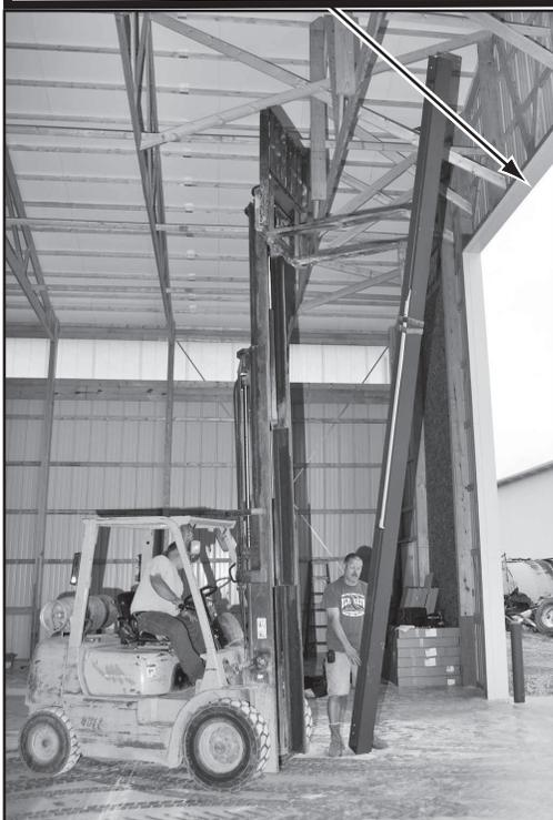
**2** [ ] Place the column into position against the door frame.
