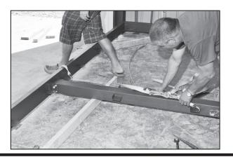
**2** [ ] If the truss is in two pieces, use four 5/8" x 2" A325 bolts for the top cord and bottom cord, and four 1/2" x 1-1/2" bolts and nuts on the web splice.
