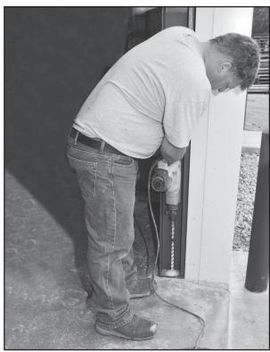
**3** [ ] As before, install another wedge anchor bolt into the other side of the slide column.
