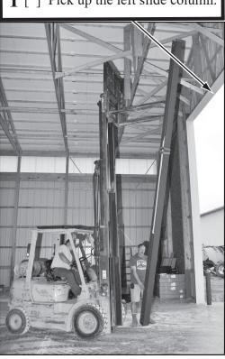
**2** [ ] Place the column into position against the door frame.
